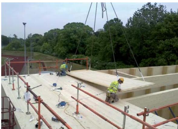
Figure 5: Installation of CLT floor panels – the construction environment is relatively free from noise and dust (Courtesy of KLH)
